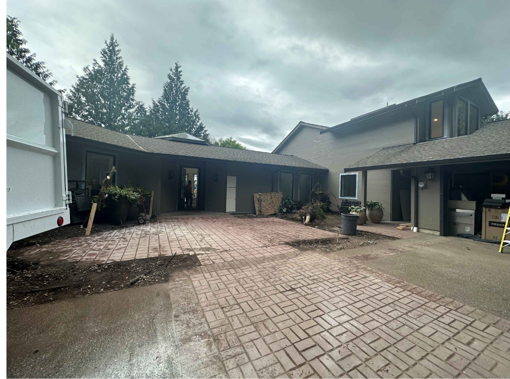
REMOVED ENTRY PAVERS
