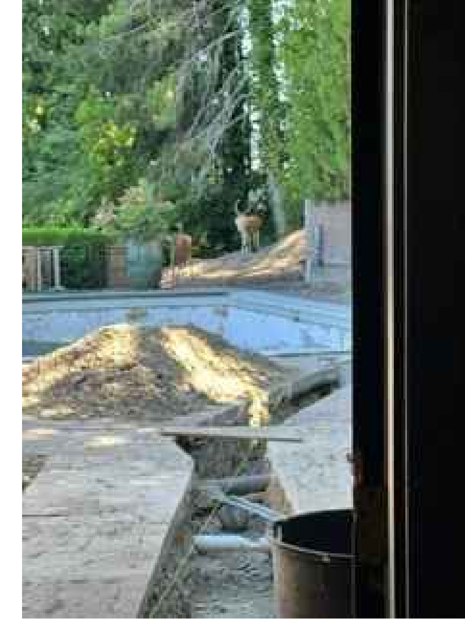
POOL AND PATIO REPAIR
